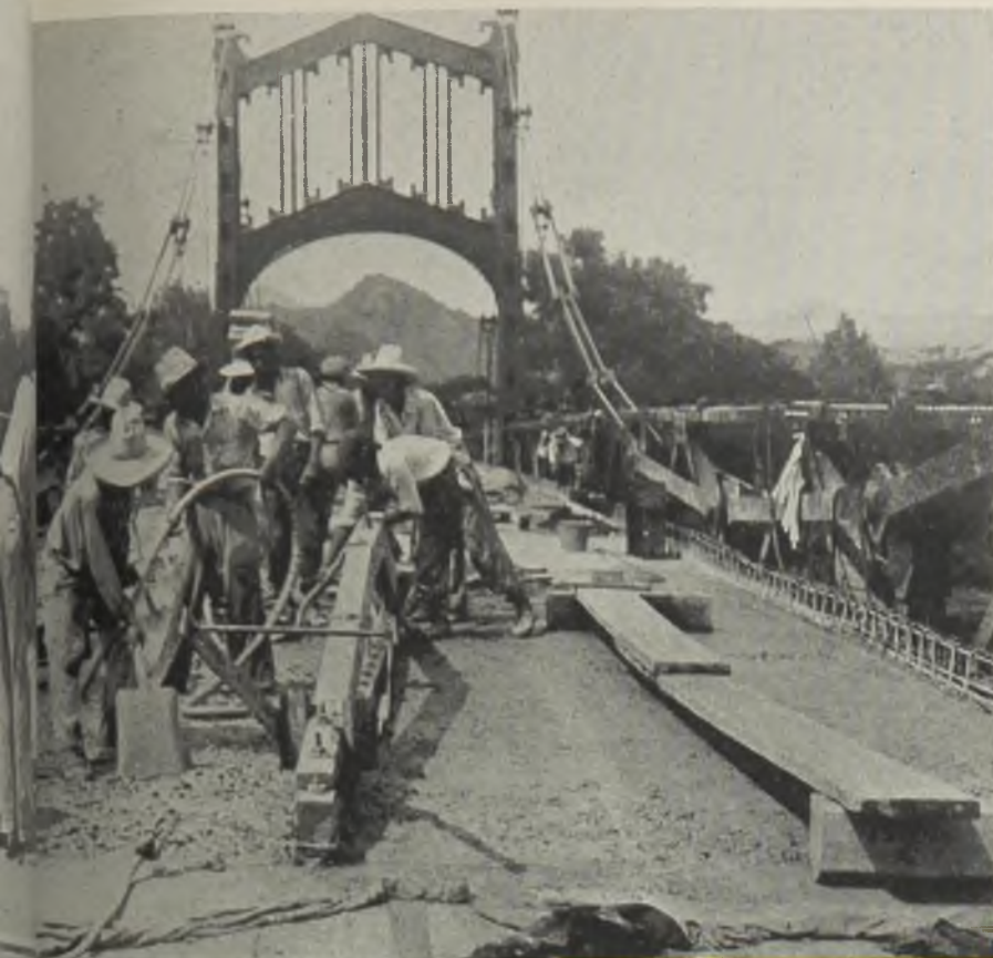
Construction view of the Tamasulpa river bridge in Guatemala, part of the Inter-American highway. Above, workmen are shown leveling concrete ahead of screed
