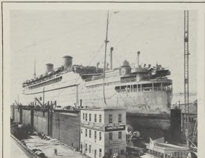
RESCUE SHIP: S. S. MONTEREY, which recently rescued 1675 of 1973 survivors of an Allied troop transport sunk in the Mediterranean, is being converted for war purposes in a Bethlehem Steel Co. ship repair yard. The War Shipping Administration praised the officers and crew of the MONTEREY for effecting the rescue while under German air attack
