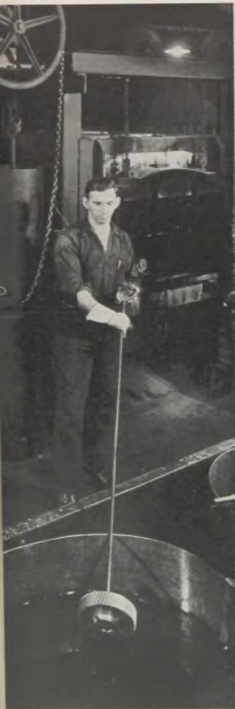
Quenching NE steel gear at National Acme
