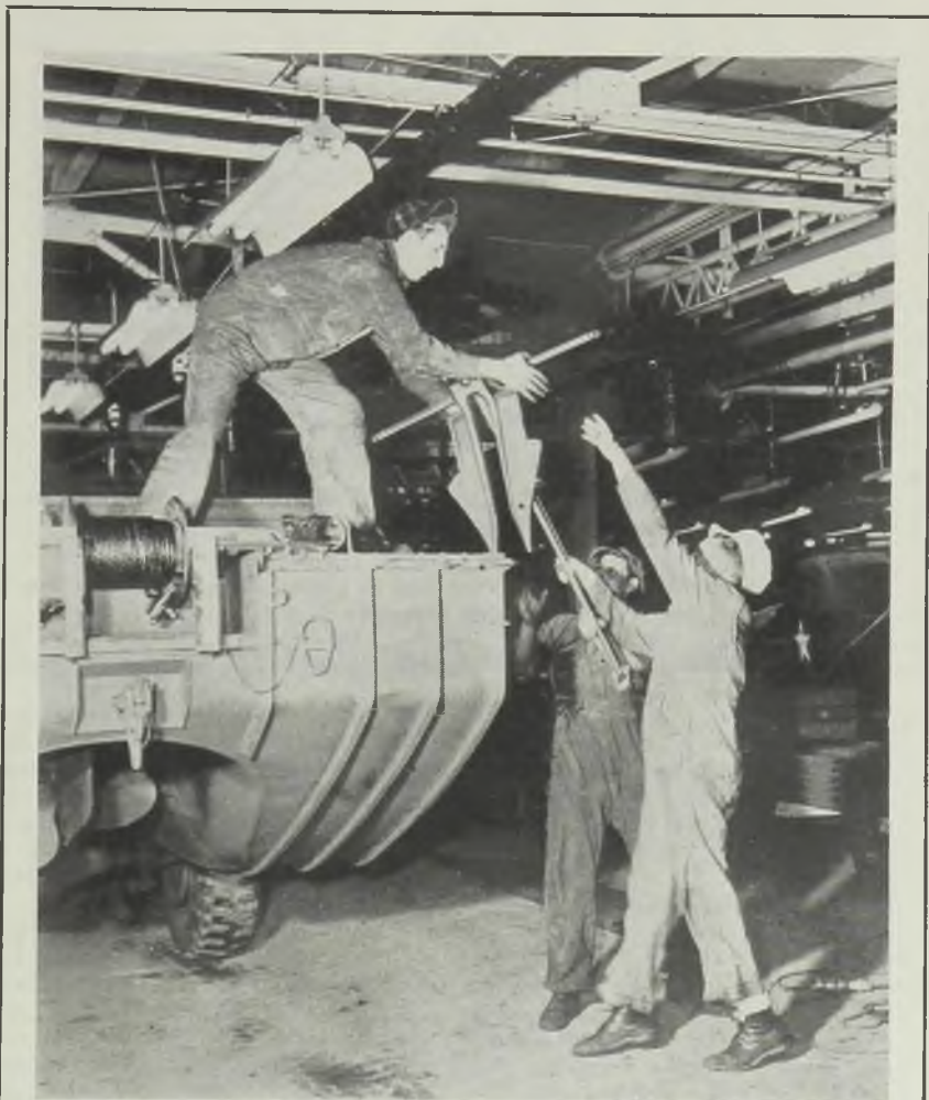
HEAVING THE ANCHOR: A novel nautical air not usually associated with an automobile assembly line is the result of the conversion of this Chevrolet line at St. Louis to production of amphibian trucks. Photo shows workers "heaving the anchor," one of the final accessories to be added to the land-water vehicle
