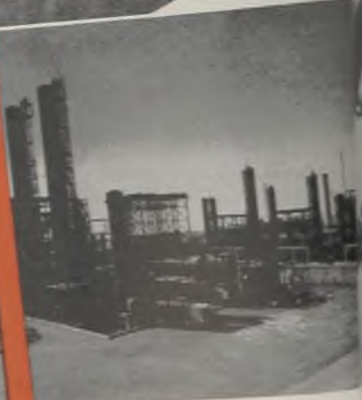
Power to win. World's largest catalytic cracking refinery for aviation fuel. Most of the pipe and tubing was NATIONAL Seamless.
