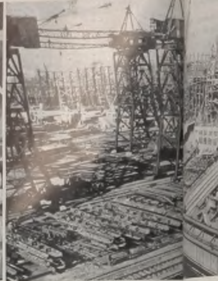
Left, workmen prefabricate ship sections in front of ways. Right, general view of an East Coast shipyard. Photos, courtesy, United States Maritime Commission
