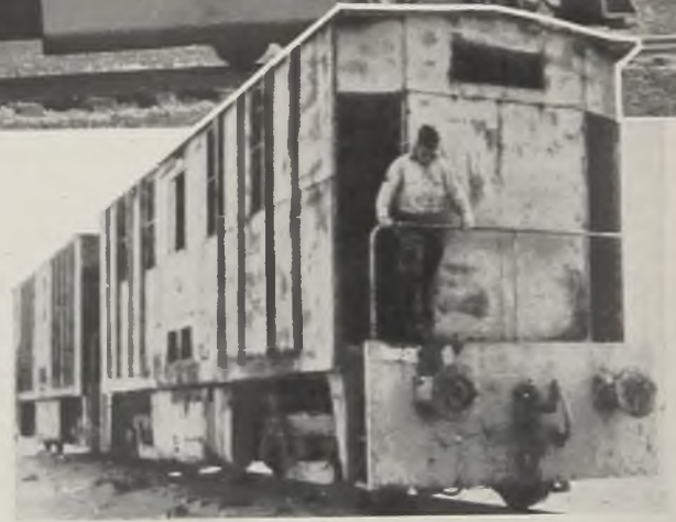
Camouflage makes this Whitcomb diesel-electric locomotive, above, look like a continental box car, right. The unit is built by a subsidiary of Baldwin Locomotive Works, Philadelphia, to transport men and materials on foreign battle fronts. The camouflage is said to be successful in deceiving enemy airmen
