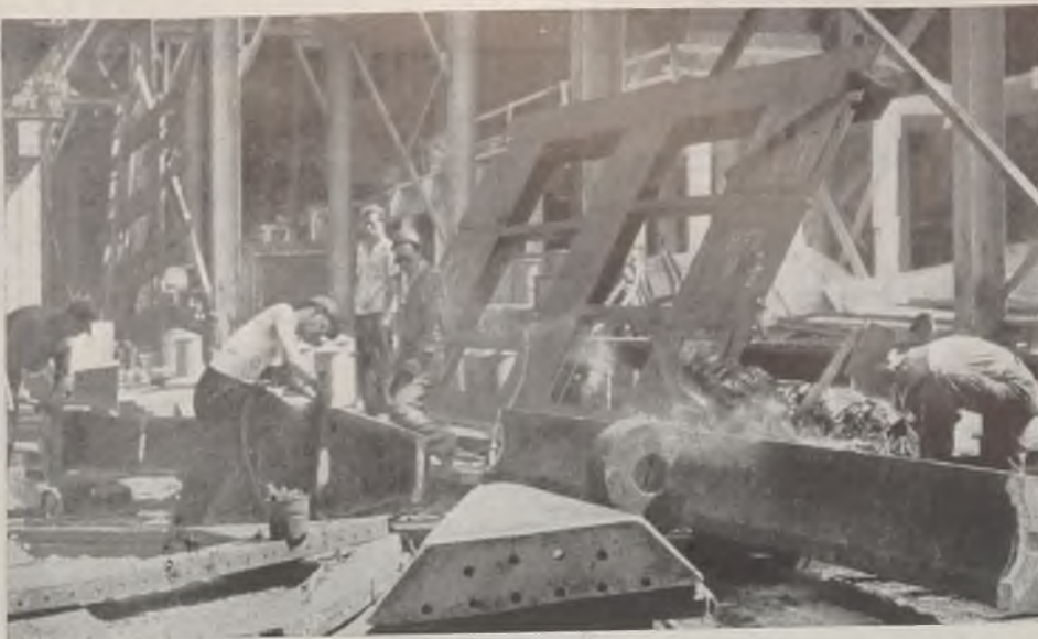
Left, workmen prefabricate ship sections in front of ways. Right, general view of an East Coast shipyard. Photos, courtesy, United States Maritime Commission
