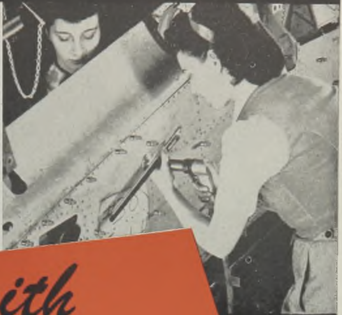
Riveting hand can be steadied while holding the RIV-N-JECTOR
