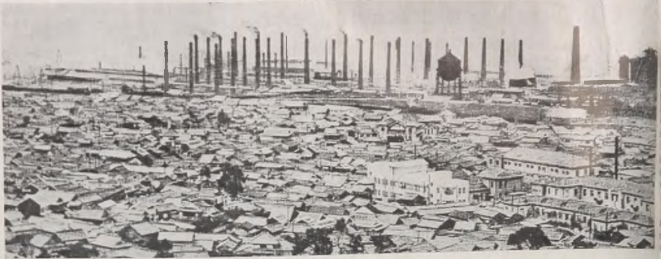
Exterior view of the Yawata steel works, recently damaged by American bombs. In the foreground are the houses of the Japanese workers. This plant is estimated to produce 80 per cent of Japan's pig iron and at least 20 per cent of its steel. Long-range B-29s struck at the heart of the enemy's steel industry. United States Navy photos from NEA
