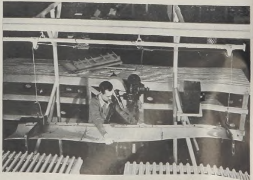
Skin panel for the forward hull bottom is riveted on an automatic riveter. Previously, all such work had to be done by hand. Note sling to enable one man to handle the large section
