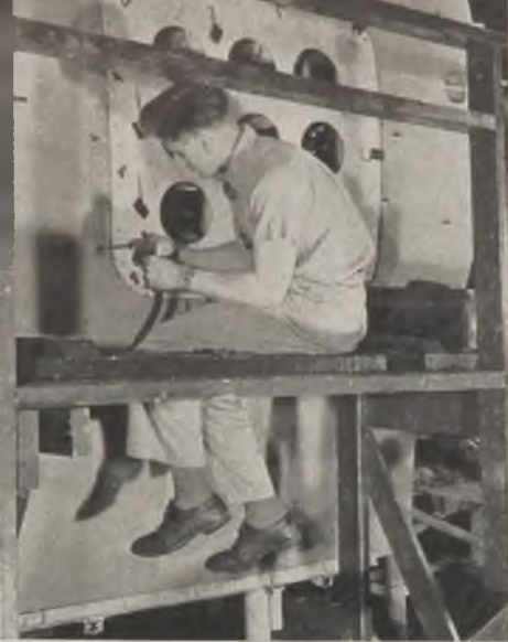
Outside strip template is used to drill the skins of the waist gunner's hatch in the aft hull section. After drilling, the skin is removed for sealing before the assembly is permanently riveted
