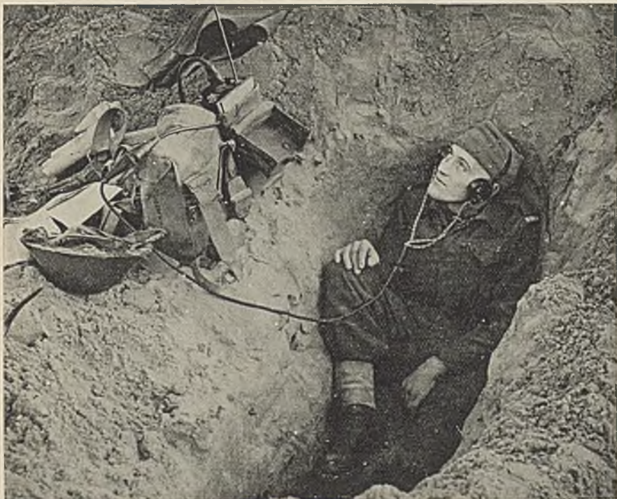
Contact with ships during landing operations. This picture was taken at Anzio. The Beachmaster's signaller dug a hole in the sand for himself and his "46 Set", and from this point he transmitted the Beachmaster's messages to the ships in the bay.
