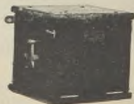
Fig. 269—Tuned Buzzer Tester.
