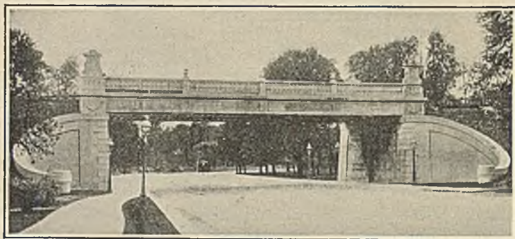
FIG. 149.—Wabash R. R. bridge in Forest Park.
