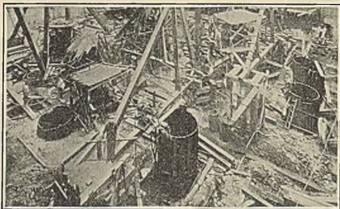
FIG. 231.—Open well foundation.
