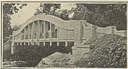
FIG. 166.—Reinforced concrete truss bridge.
