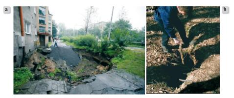
Figure 1. Examples of discontinuous deformations: a) local collapse (http://bi.gazeta.pl/), b) crevice (own archive)
