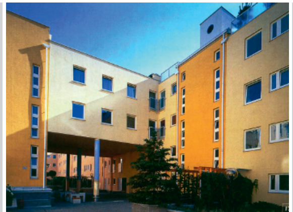
Figure 2. Oaza Colony, Warsaw, ul. Białobrzaska, (designed by: K. Kucza-Kuczyński, J. Kucza-Kuczyński, M. Krauze, A. Miklaszewski), fragment of the inner courtyard with the connecting wing. Source: "Architektura-Murator" no 12, 2003, p.34, Photo: D. Rumiancew
