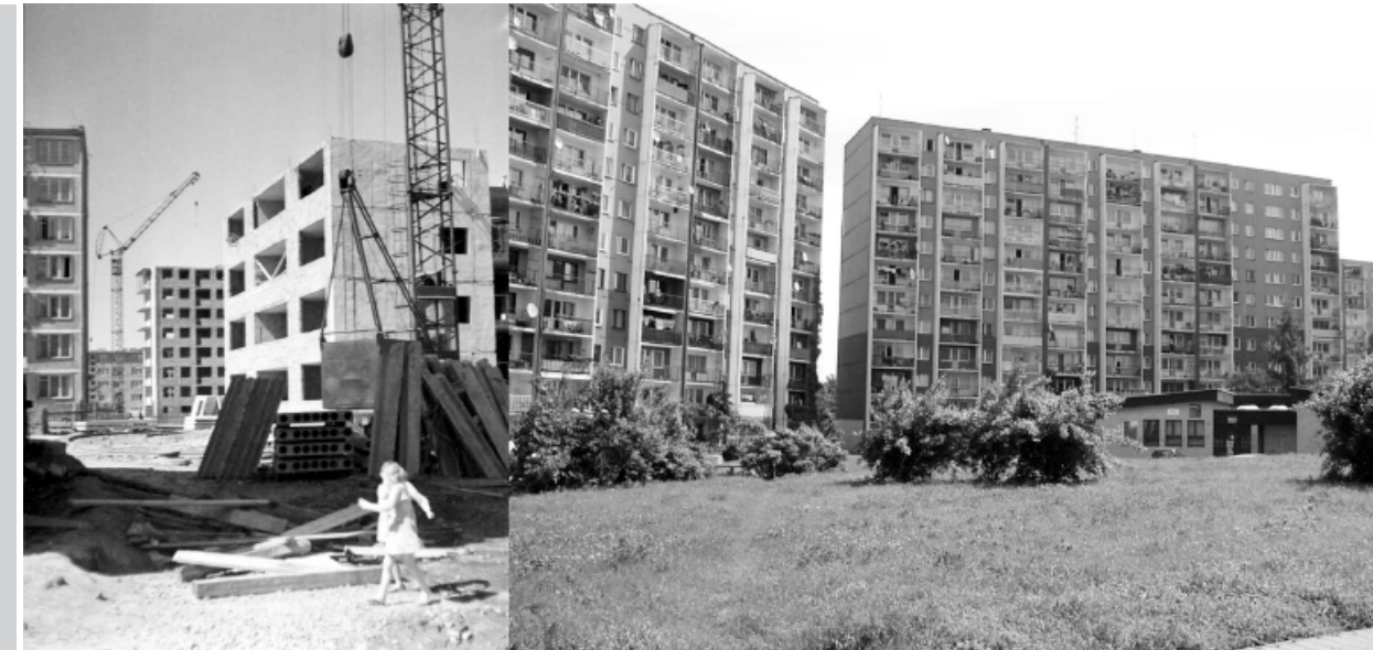
Figure 3. Slab technology houses in Tychy and Gliwice, erected in 1970s
