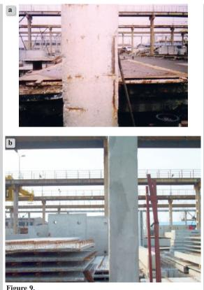
Reinforced concrete columnar structures: a) corroded concrete reinforcement, b) after renovation
