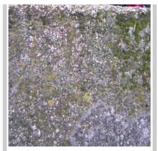
Figure 1. Concrete foundation covered with different lichens
