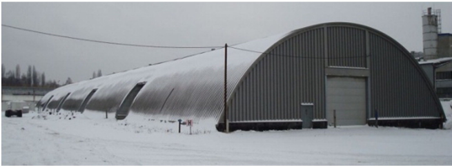
Fig. 5. Warehouse constructed in ABM 120 technology.
