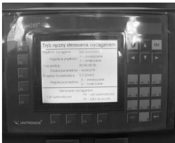
Fig. 2. View of control panel
