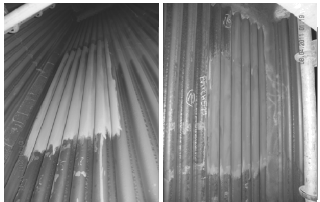
Fig. 10. The coating with sealing process on the components of power boilers
