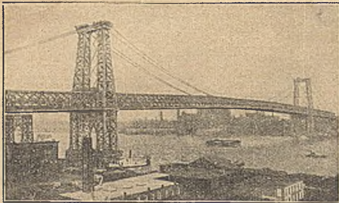
Rys. 2. Most Williamsburg Bridge na East River w New Yorku
