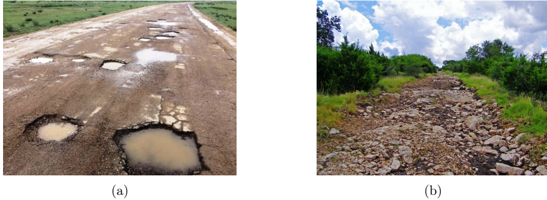
Figure 1.1: Examples of road-induced excitation of vehicle vibrations: a) single-road-bump excitation; b) continuous excitation
