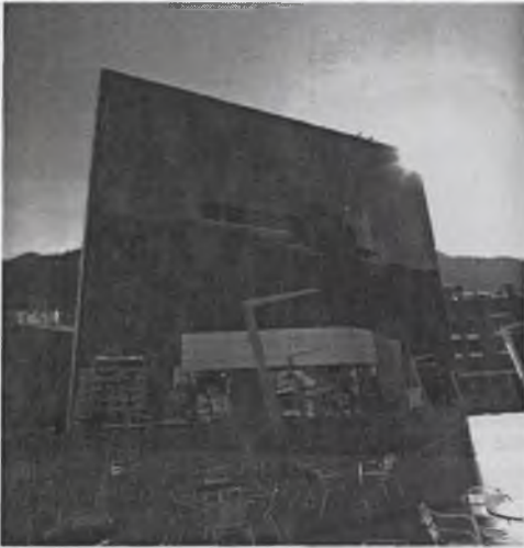
Fig. 3. General view of Encamp Town Hall, photo by Francesco Tur [3]
