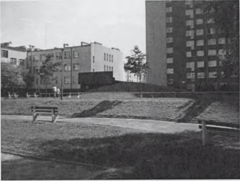
Rys. 5. Hydrofor Fig. 5. Water-supply system
