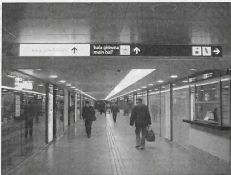
Rys. 1. Podziemia pod Dworcem Centralnym w Warszawie, stan po remoncie. Fot. K. Juchnevic Fig. 1. Underground AT the Central Station In Warsaw, the state after repairs. Photo K. Juchnevic
