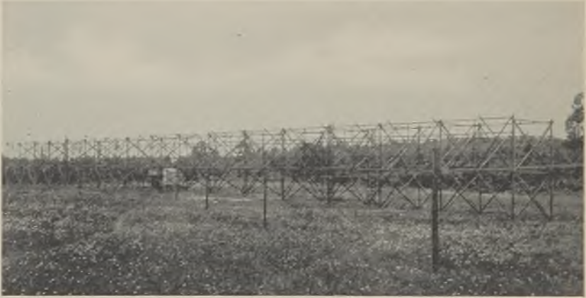
Fig. 18—Bruce receiving antenna at Netcong, New Jersey, used for transoceanic communication. This type of antenna has been superseded by the rhombic type at Netcong.
