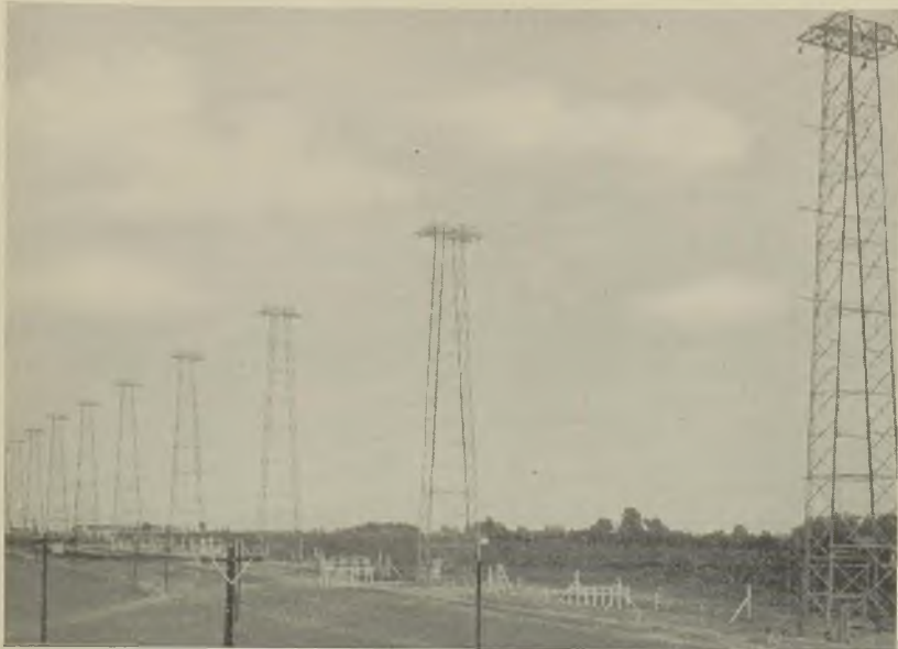
Fig. 16—Towers at Lawrenceville, New Jersey, used to support a number of Sterba antennas for transoceanic communication. These antennas have since been superseded by rhombic antennas.
