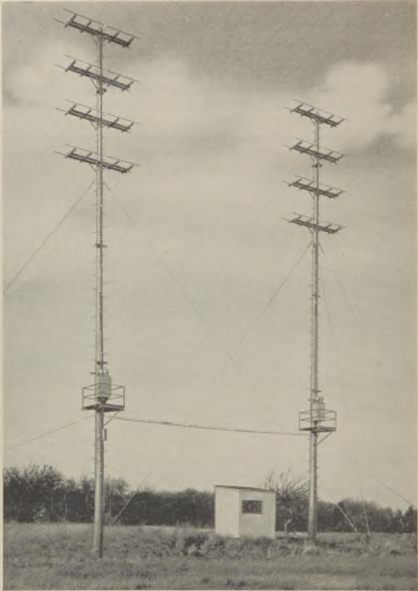
Fig. 20—Pine tree antennas used on Provincetown-Green Harbor ultra-short-wave circuit.
