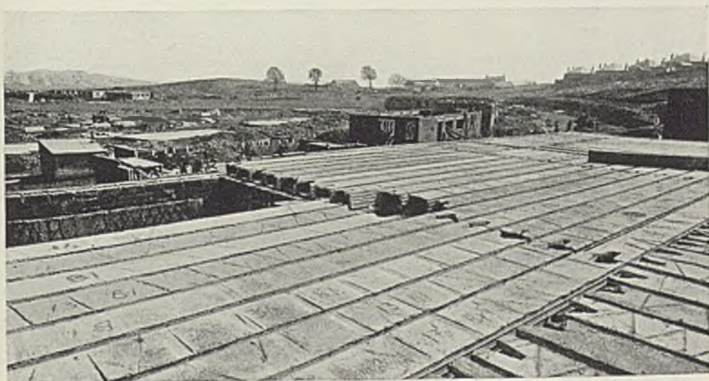
Figs. 143, 144. Constructional views of houses, Penilee Estate
