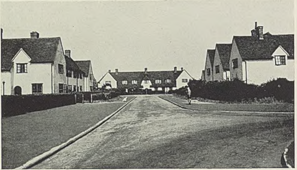
FIG. 98. A quiet corner amongst working houses
