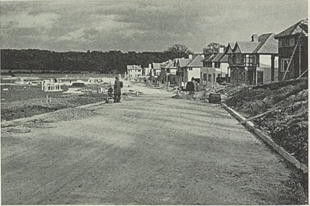
FIG. 22. A concrete road affords easy access to building sites
