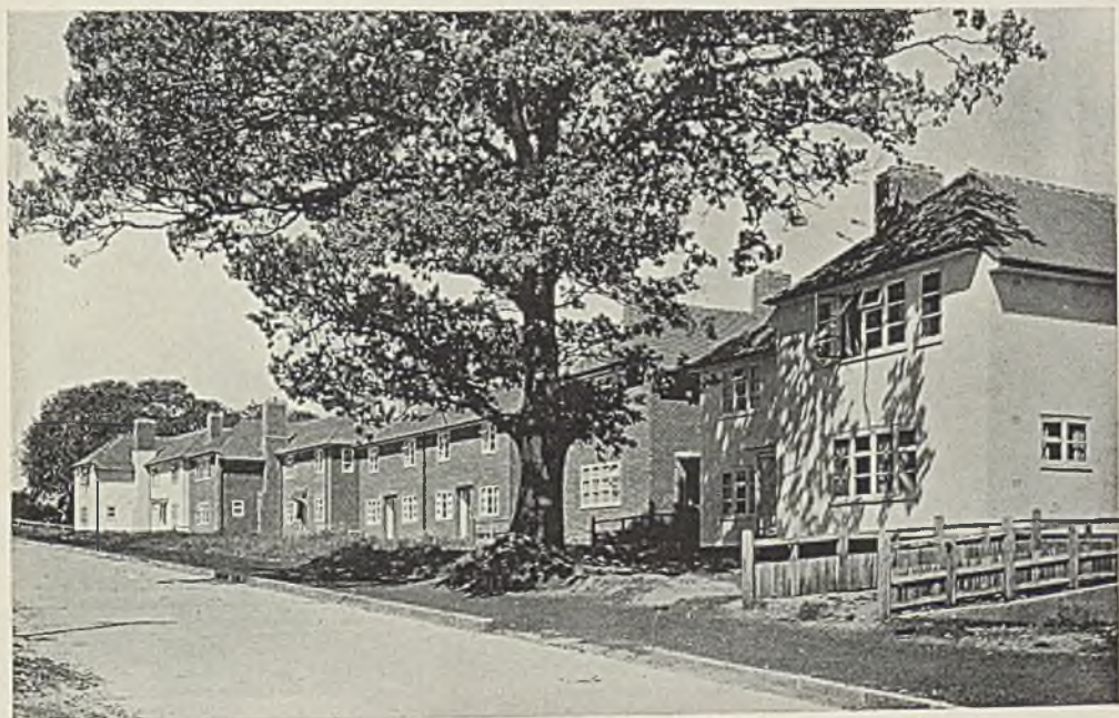
FIG. 130. Parlour type houses, Lea Hall Estate BIRMINGHAM
