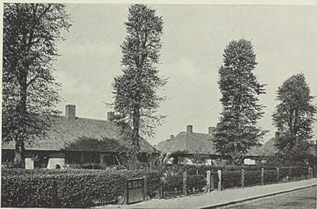
FIGS. 162, 163. Brick bungalows, Wollaton Park Estate NOTTINGHAM
