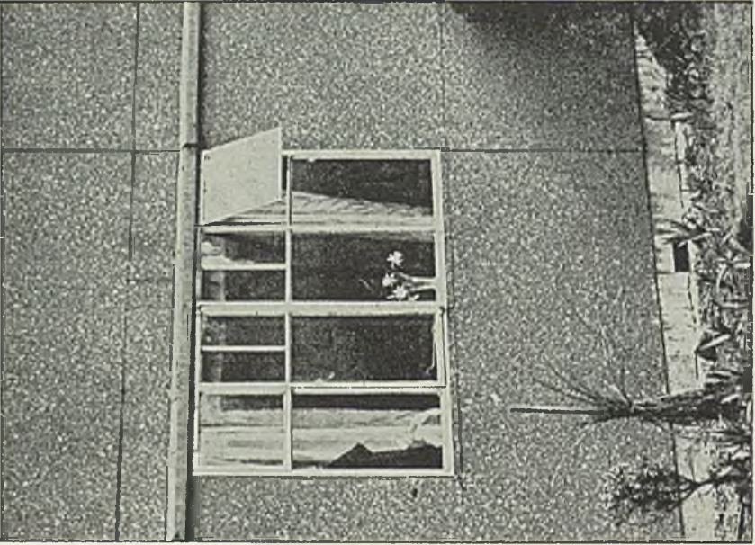
FIG. 44. Jointing of sheets in the Weir house
