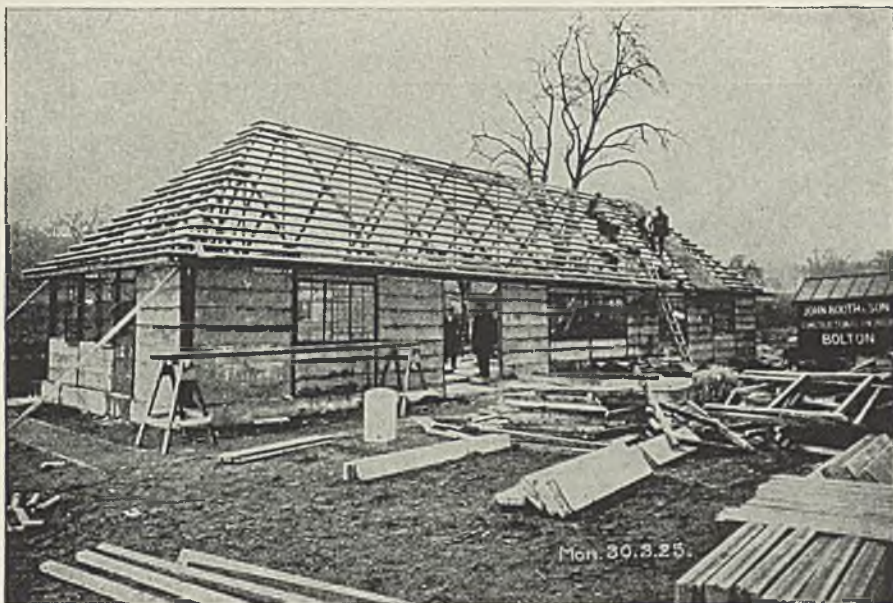
FIG. 41. The Crane house in construction
