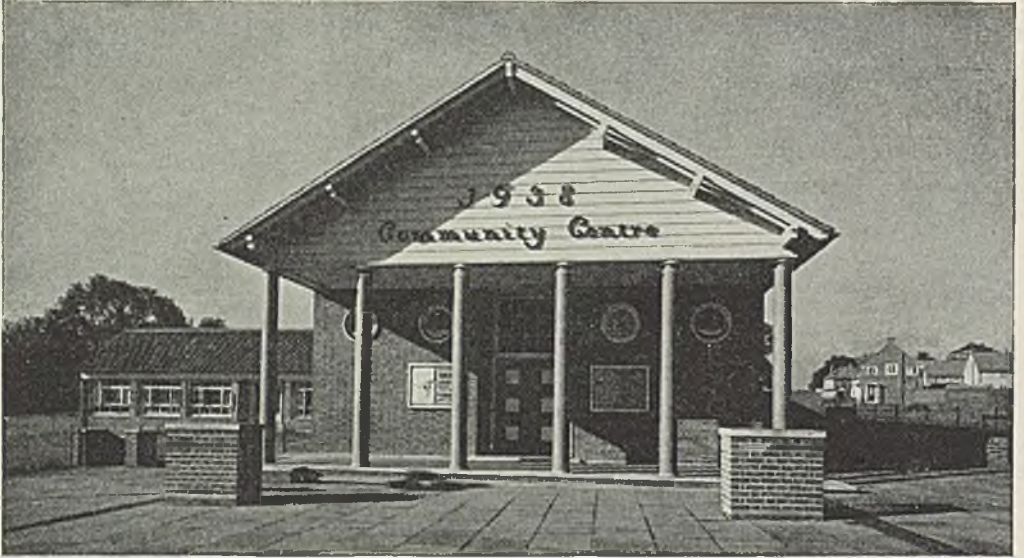
FIG. 105. The community centre
