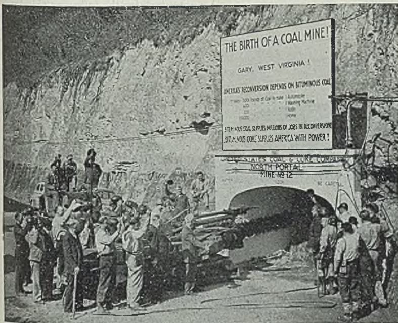
COAL MINE IN THE SKY: A new bituminous coal mine atop a mountain 2200 feet above sea level is being opened at Gary, W. Va. A cutting machine makes first cut in the exposed coal seam 9 feet thick over which a concrete portal has been built. Mine is estimated to produce 250,000 tons a year
