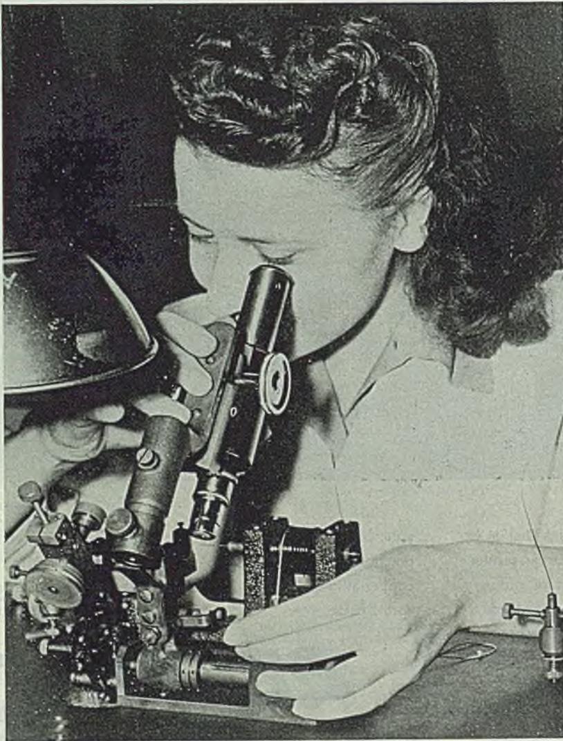
DRILLING DIAMONDS: A microscope is necessary to check progress in drilling a diamond die, a slow process which takes from 3 to 9 days. Proper shape of those dies made by North American Phillips Co. Inc., New York, is essential for drawing high-quality fine-wire products to be used in electronic devices
