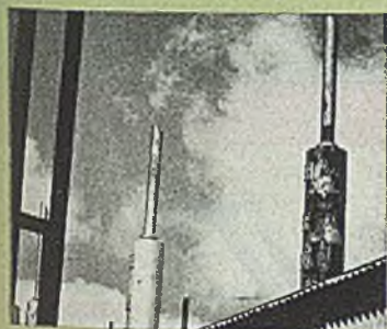
The excellent condition of the stack at left, protected with silicone based paint, indicates the ability of such finishes to withstand moisture, oxidation, ultra-violet rays and temperatures up to 500°F.
