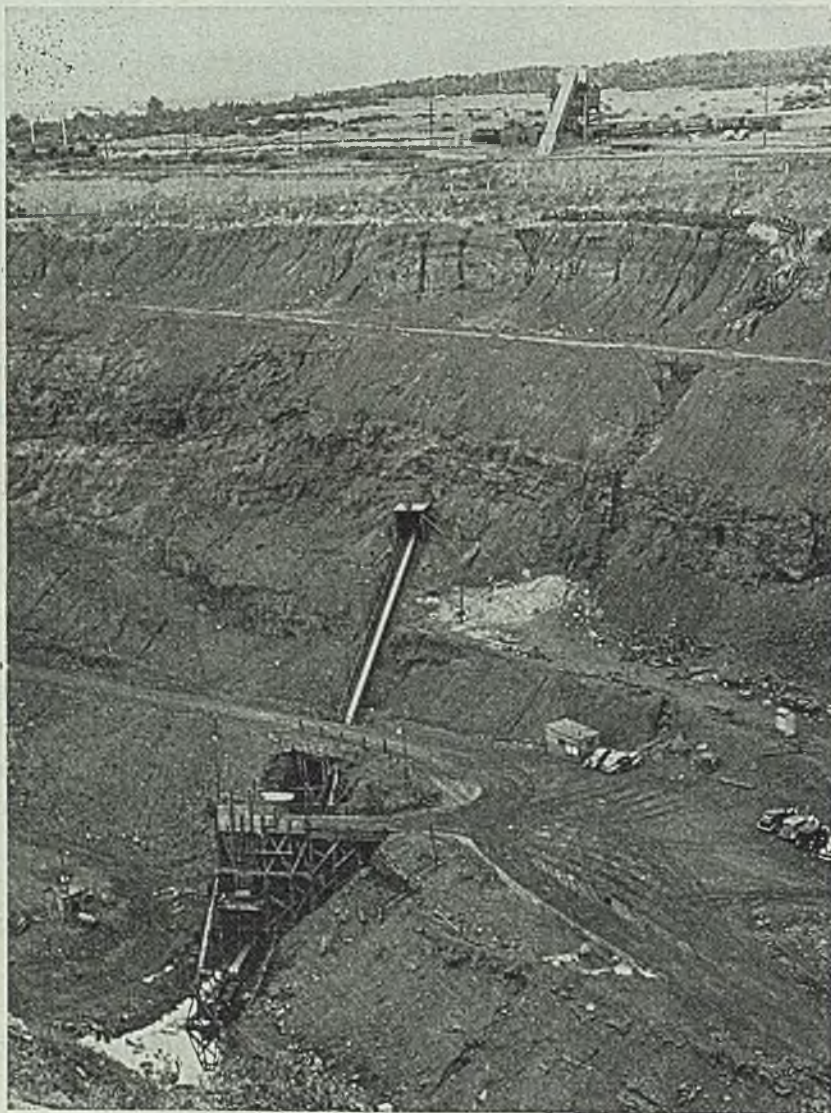
LONG LIFT: Believed to be the greatest lift made by any single conveyor belt in the world, this cord construction ore carrier made by B. F. Goodrich Co. is 1900 ft long, 30 in. wide, and center-to-center distance is 947 ft. Total lift is 272 ft, grade is 35.53 per cent, and speed is 578 fpm. Belt handles 550 tons per hr of wet or dry ore, and in its first year of operation handled 1,250,000 long tons of ore and saved $15,000 in transfer and maintenance costs required by the previous three-belt installation, at Missabe Mountain pit of Charleston Iron Mining Co. in Minnesota
