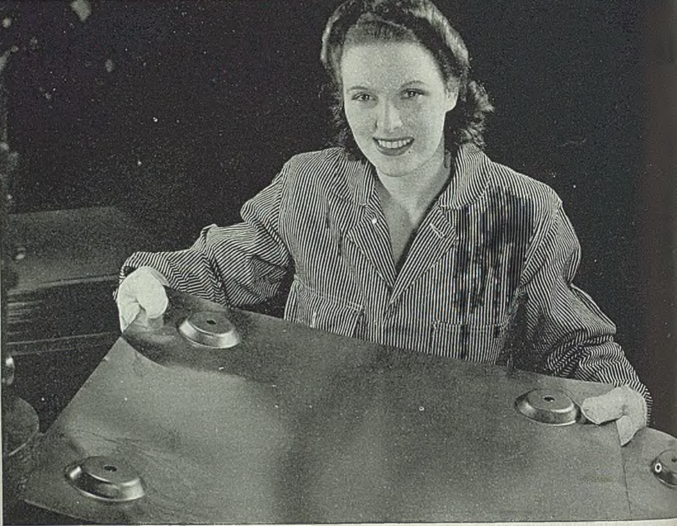
Forming pockets in Inland sheets is the first operation in making heads for 5-gal. containers.
