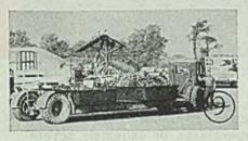
Fig. 8—Manually operated hydranlic lift trucks handle assortments of finished small parts being moved from storerooms to assemblu on accumulating trays pictured here
