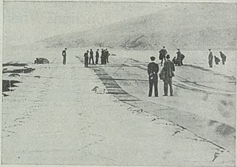
OCEAN LANDING STRIP: British Admiralty has developed airplane landing strips for use on the surface of the ocean which will accommodate planes loaded up to 9000 pounds. The strips are made of hundreds of hexagonal cans so assembled that the motion of waves provides tension for a heavy canvas surface. NEA photo
