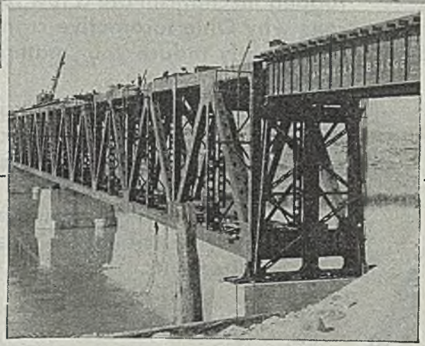
The new, high-level Topock Bridge replaces an old through-truss cantilever crossing Colorado River. The old bridge (not shown) is located at the extreme right end of the alignment of the low-level roadbed in the foreground. The new, ballasted-deck structure consists of three, 370-foot deck truss spans over the main channel with plate girder spans to the east and west, respectively 150 and 300 feet long. The steel superstructure was designed and erected by American Bridge Company.
