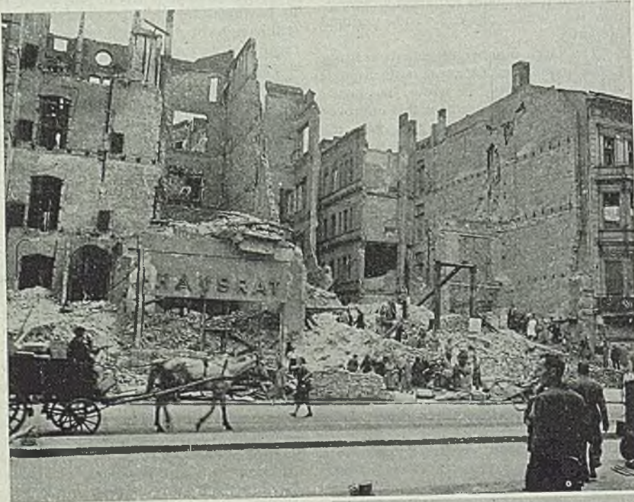
Bucket brigades of women clean up rubble in Berlin, above. A lack of modern reconstruction program in Germany, formerly one of the most highly mechanized countries of the world, is one of the paradoxes of the war. At right is a wrecked oil refinery at Hamburg
