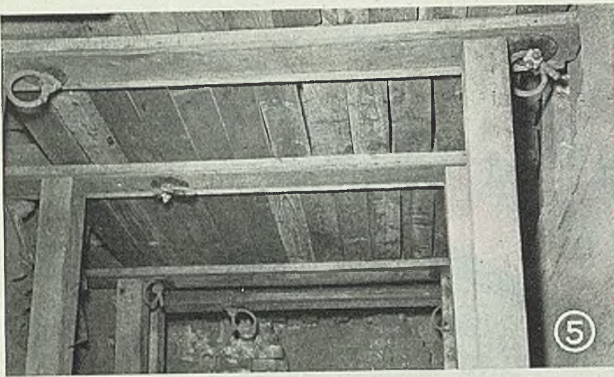
Fig. 5—How roof was installed to protect workmen
