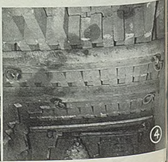
Fig. 4—Oak timbers and cables that were employed to support the furnace checkerwork
