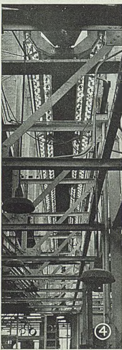
Fig. 4—View of Hayes Industries infra-red oven shows how it was mounted high in the building structure, thus saves $2880 monthly in floor space; at same time, output was tripled
