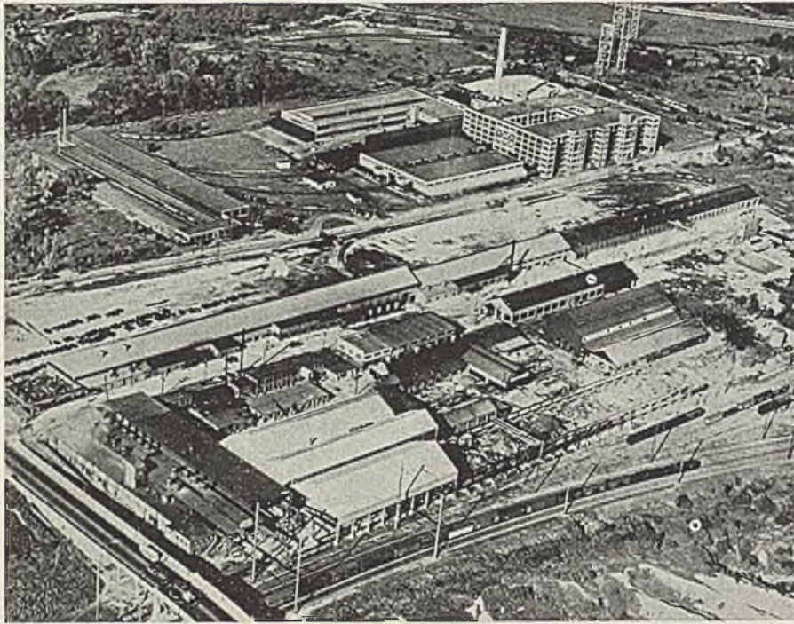
Works of the Rustless Iron & Steel Corp., one of the leading producers in the Baltimore area, as seen from the air. Company produces stainless steel semi-finished, bars, rod and wire. NEA photo
