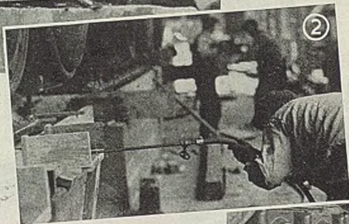
Fig. 2—Top of foundation and bolt holes are suction cleaned
