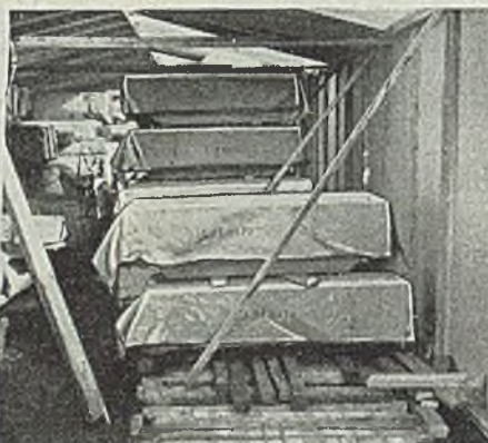
Temporary emergency storage shelters are made with Fibreen on 2"x4" frame.
