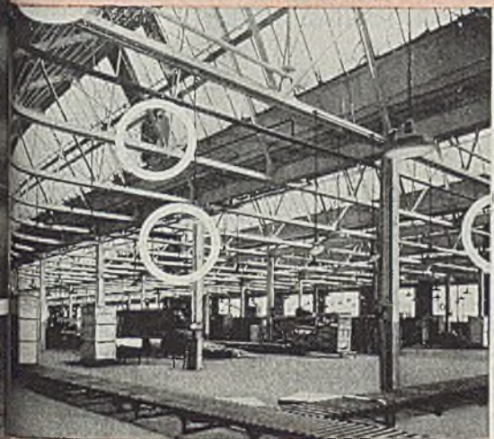
ASSEMBLY PLANT with high saw-tooth roof conserves heat when Speed Heaters are strategically located in accordance with size and shape of the area, proper paths of heat travel.
