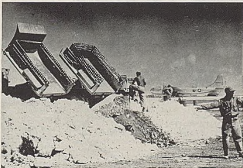
SPEEDING THE JOB: American Seabees increased the capacity of their dump trucks by adding airway matting to the beds of the trucks, permitting them to haul larger loads of crushed coral used in building runways for B-29s at a Guam base. NEA photo
