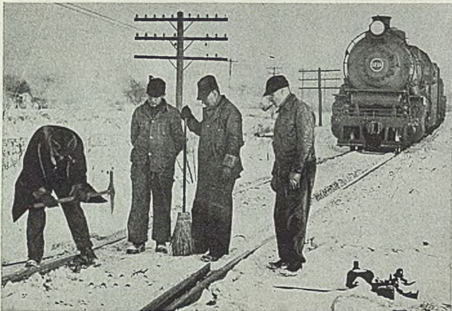
Line engine waits in the Bedford, O., yard of the Pennsylvania railroad while track workers spike a switch in reverse so it can enter the yard. Photo by Yassenye, Cleveland Plain Dealer
