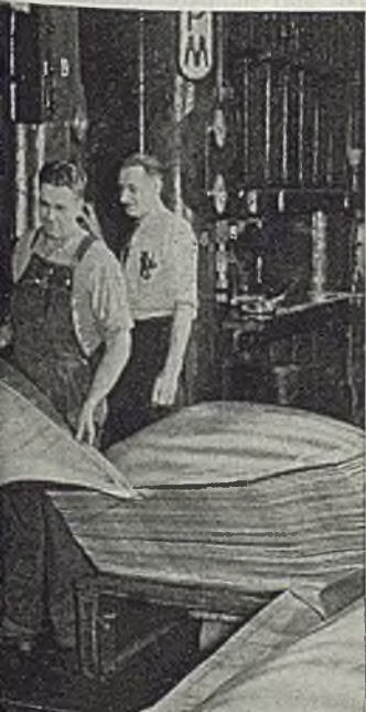
Fig. 4—Typical of the equipment in the huge press shop at Ford's Willow Run plant is this row of stamping presses. Unit in foreground is 275-ton capacity press being used to stamp out a spar which goes in the fin of the empennage of the Ford-built Liberator. This press was moved from the Rouge plant to Willow Run along with other equipment when bomber job was started
