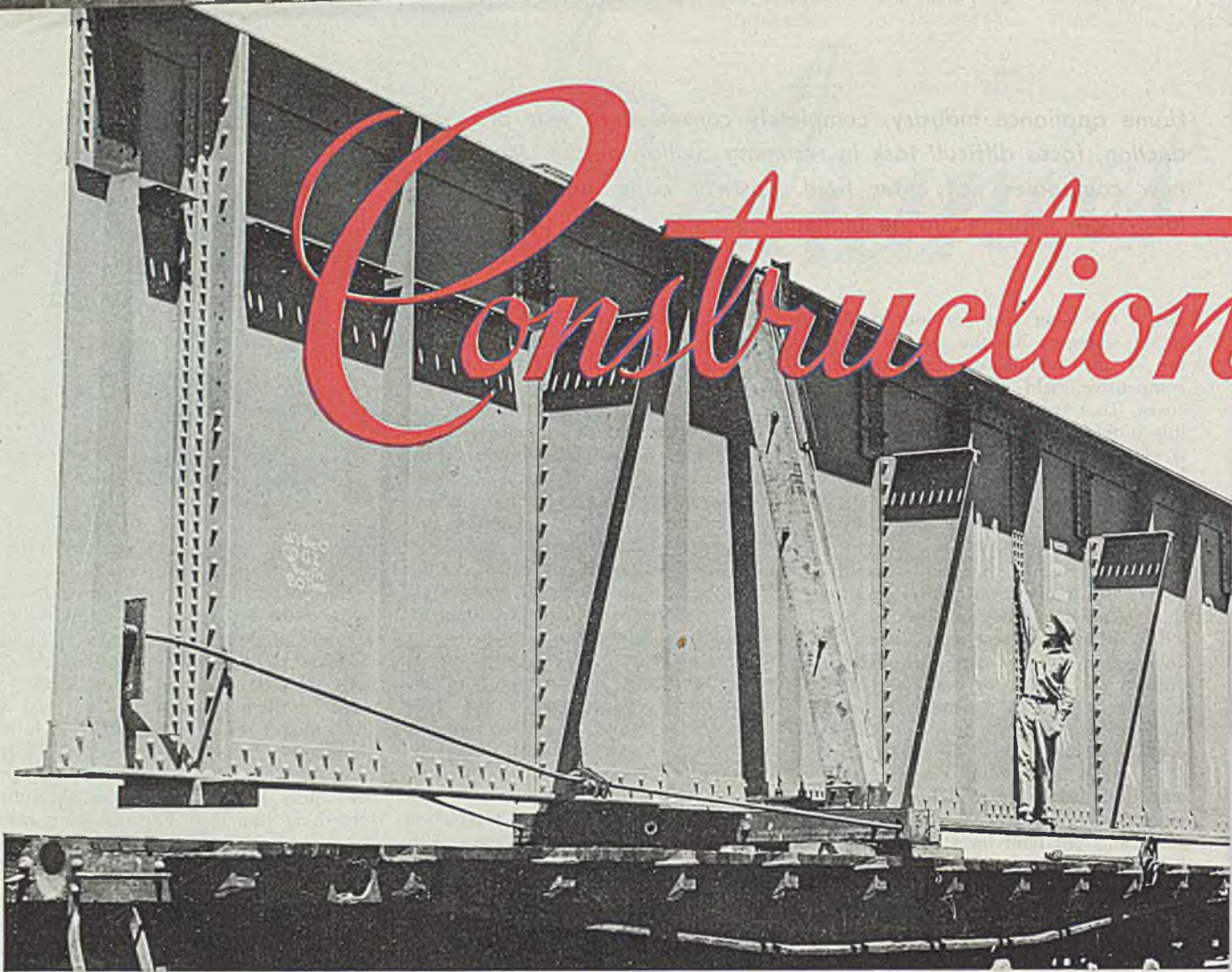
One of the largest pieces of fabricated steel ever to be transported by rail, this bridge girder required three flat cars equipped with special couplings and support plates to distribute the weight. The girder is 154 feet long, weighs 97 tons. NEA photo
