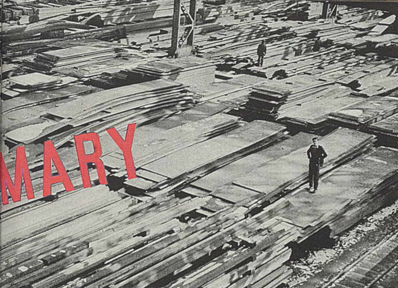
View in receiving yard of the Ambridge Works, American Bridge Co., U. S. Steel subsidiary. These plates, angles, channels and other structural steel units are ready to be placed in fabrication when needed
