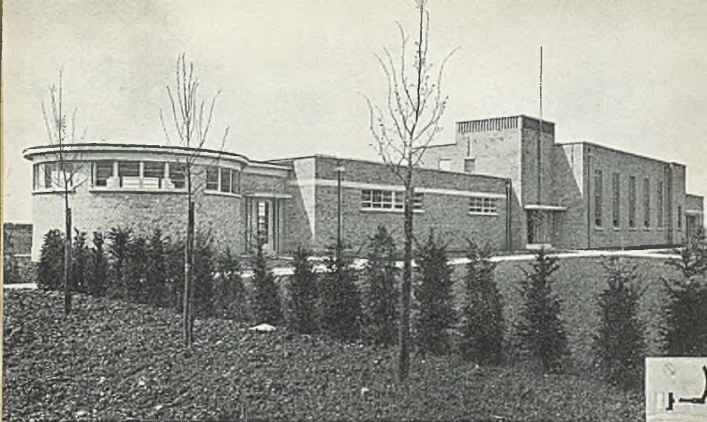
BOTTISHAM VILLAGE COLLEGE, CAMBRIDGE (Architect: S. E. Urwin) One of the 'village universities' resulting from the genius of Dr. Henry Morris, Director of Education for Cambridge, which are giving a new dynamic impulse to life in isolated small communities
