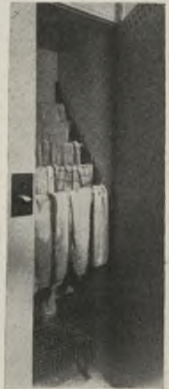
Drying cupboard with heating unit at base
