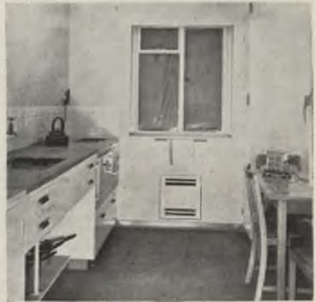
No. 3 kitchen with heater under the window
