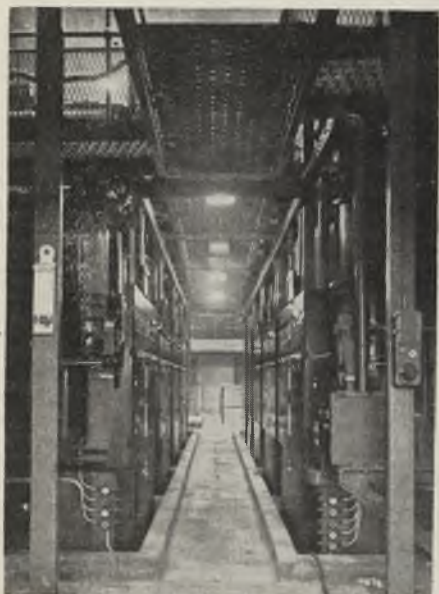
33 kV, 1 500 MVA switchgear
