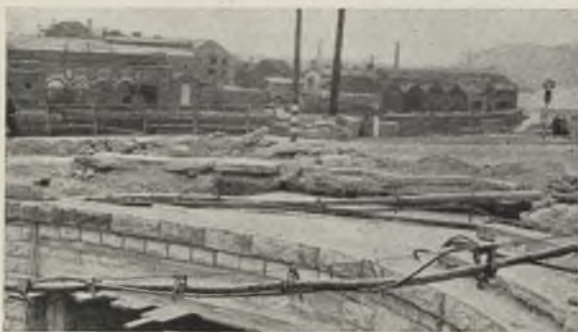
An expedient for supporting temporary cables alongside a damaged bridge
