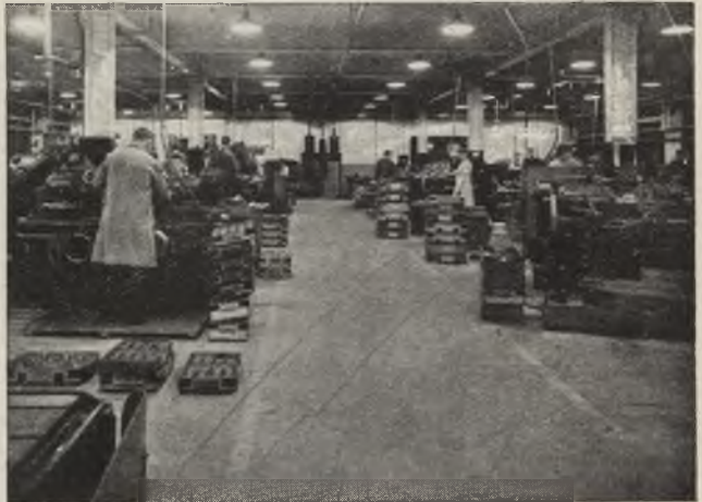
A new B.T.H. lighting scheme for a machine shop
