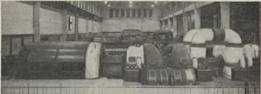
The four 30 000 kW English Electric turbo-alternators
