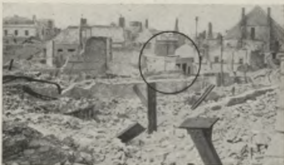
The only building left standing in this area was the sub-station shown in the circle
