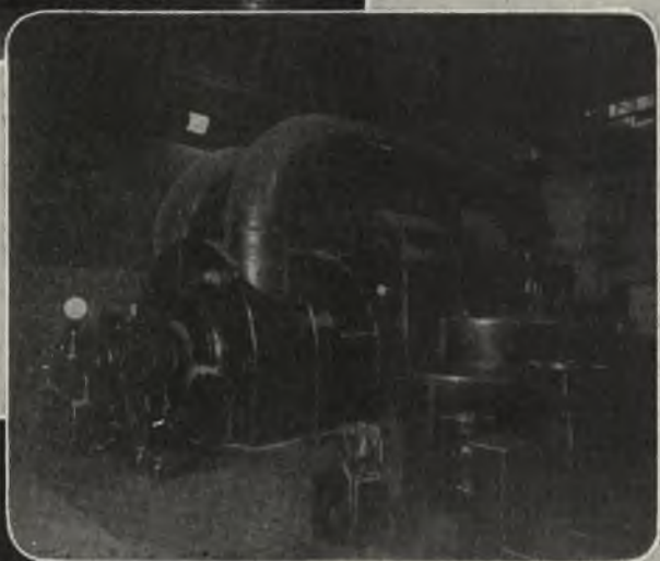
Right:—The B.T.H. 60 000 kW turbo-alternator
