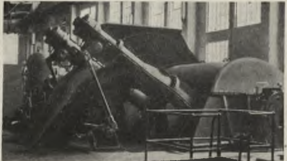
Part of English Electric hydro-electric plant installed in Tasmania
