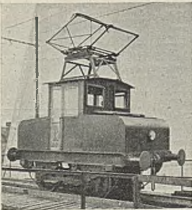
Fig. 1.—Standard gauge electric loco' supplied by the English Electric Co., to Sunderland electricity department
