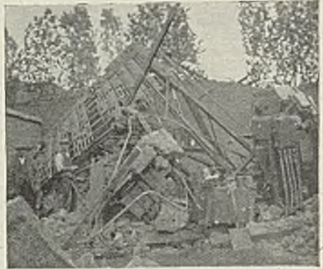
Sub-station demolished by a direct hit at Battersea
