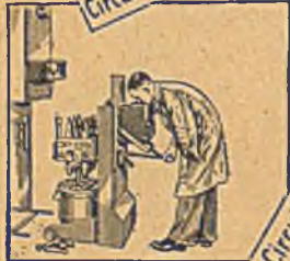
Circuit Breaker Truck withdrawn from cubicle
