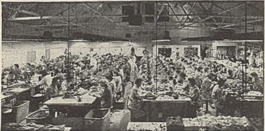
Osram fluorescent lighting in a clothing factory
