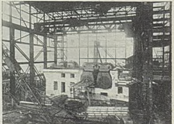
Turbine block with both halves of condenser in position at July 8, 1942
