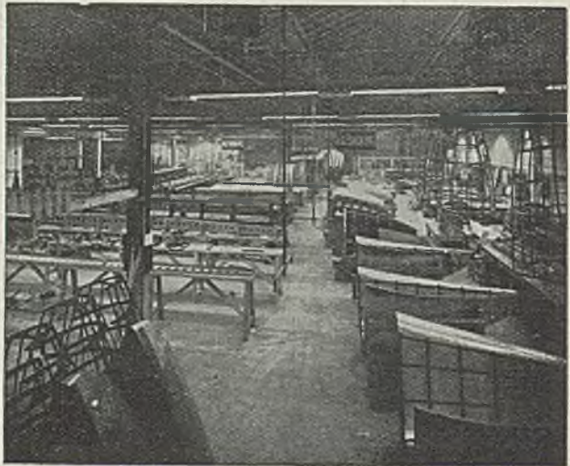
Fluorescent lighting in a Manchester works
