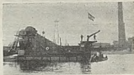
Cable-laying on the River Weser 38 years ago
